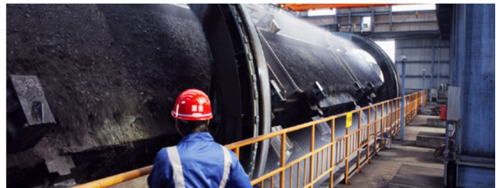
Material handling: Railcar dumper and positioner systems
