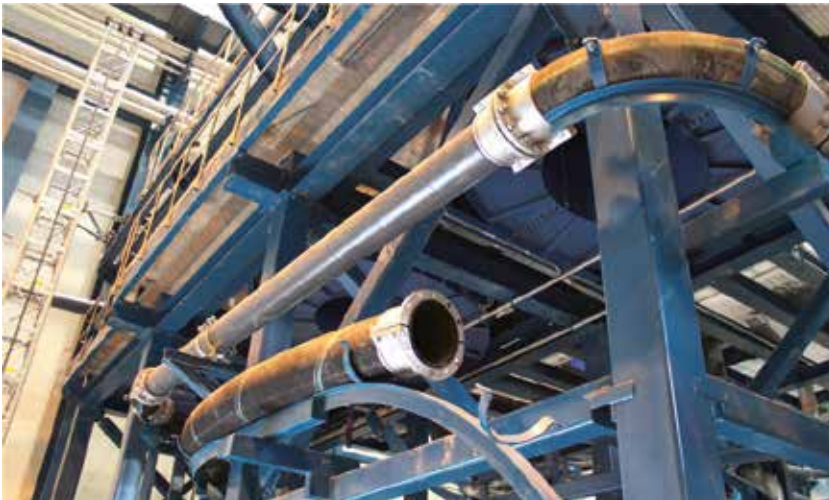
Picture 3: Material handling hose, rubber lined steel pipe, 3x90 Degree bend and support clamps
