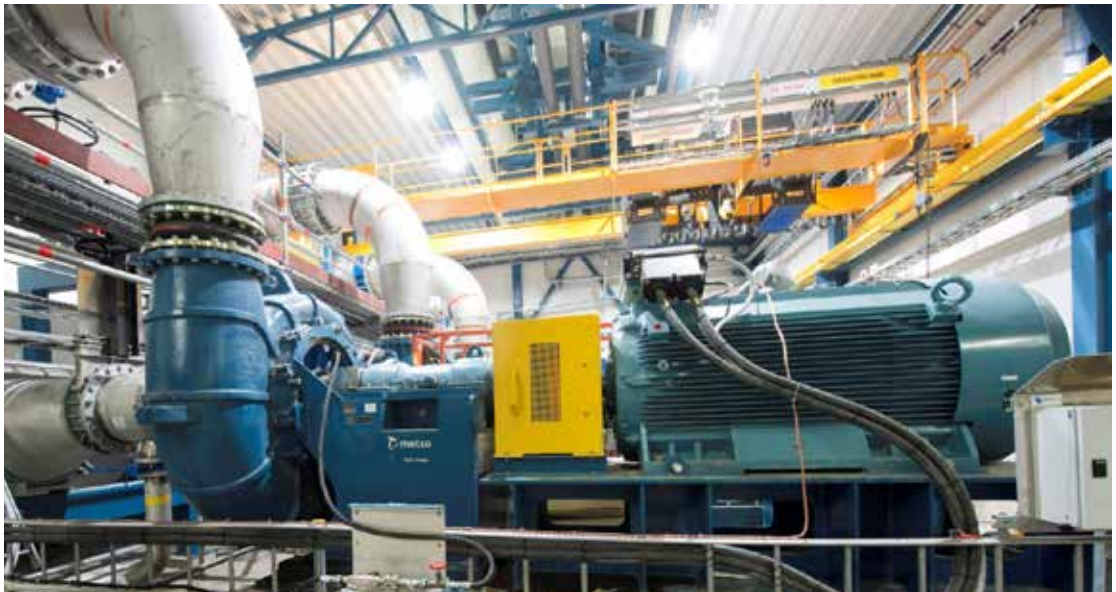
MM pump with direct coupled motor
