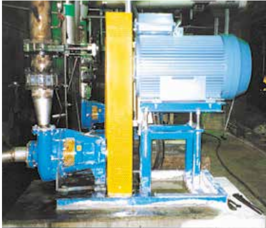
HM pump with reverse overhead mounted motor and v-belt drive.
