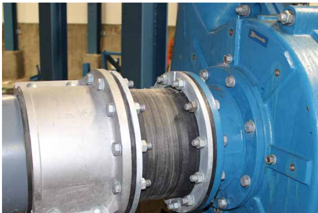
Picture 5: Rubber lined steel pipe and compensator
