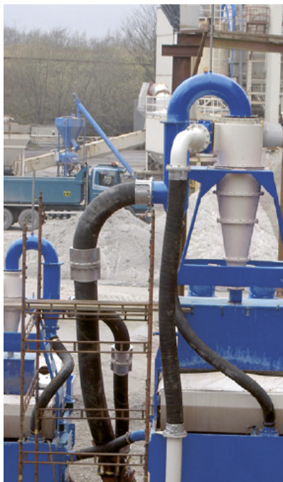
Picture 4: Material handling hose with 3xD 90 degree bend
