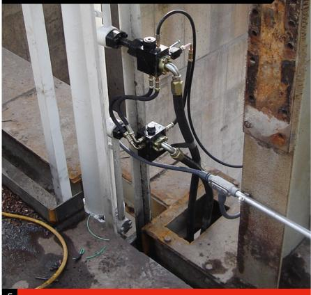
Options include raising dumper drive units to track level, converting to dual drives, installing a spindle operated dumper latch, relocating hydraulic manifolds, moving hydraulic power units off board and more. Improve your safety and availability with drive and hydraulic upgrades.
