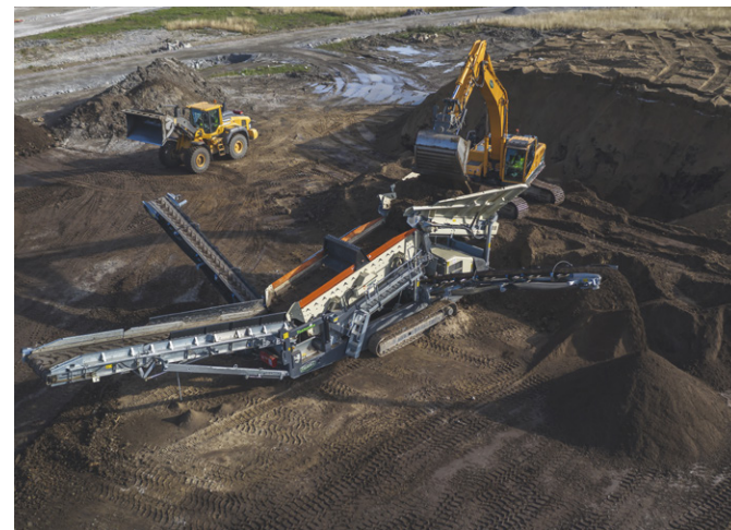
Crushing and screening of overburden
