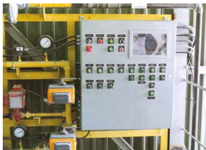
Typical burner management system
