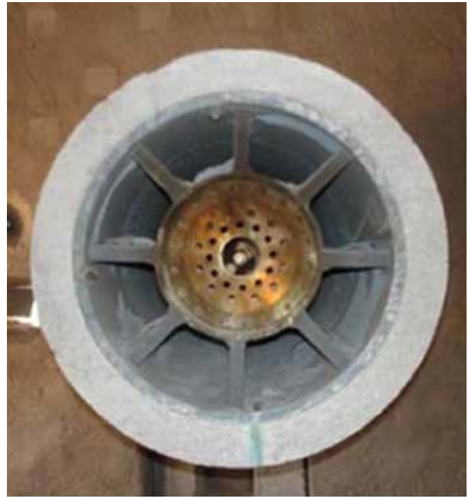
A typical pulverized fuel/gas burner
