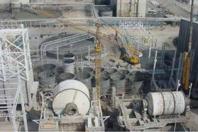
Conditioners and surge tanks Slurry Pumps, Slurry Piping
