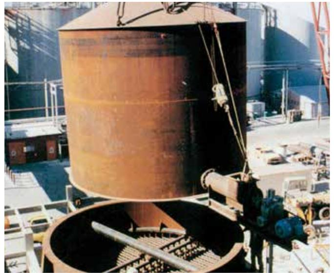
*Steam heated aluminum hydrate fluid bed dryer.*
