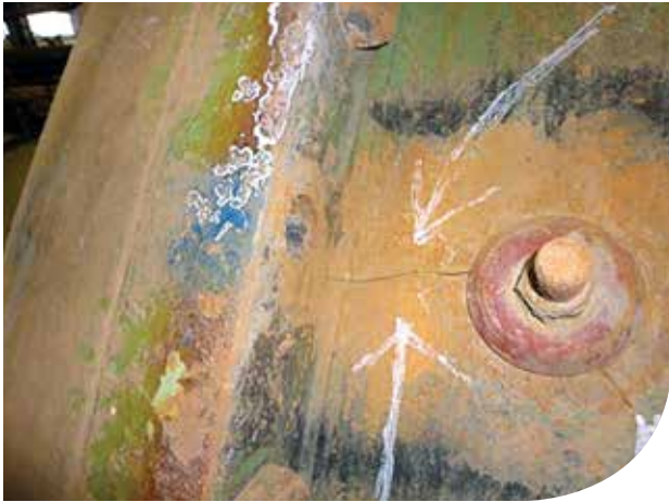
Mill Visuals and Vitals: An external crack discovered on a mill shell while performing a visual inspection.
