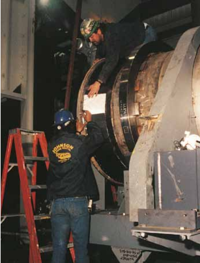
Superdeal kiln seal in the final stage of installation.
