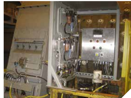
An infrared temperature system tracks the readings continuously
